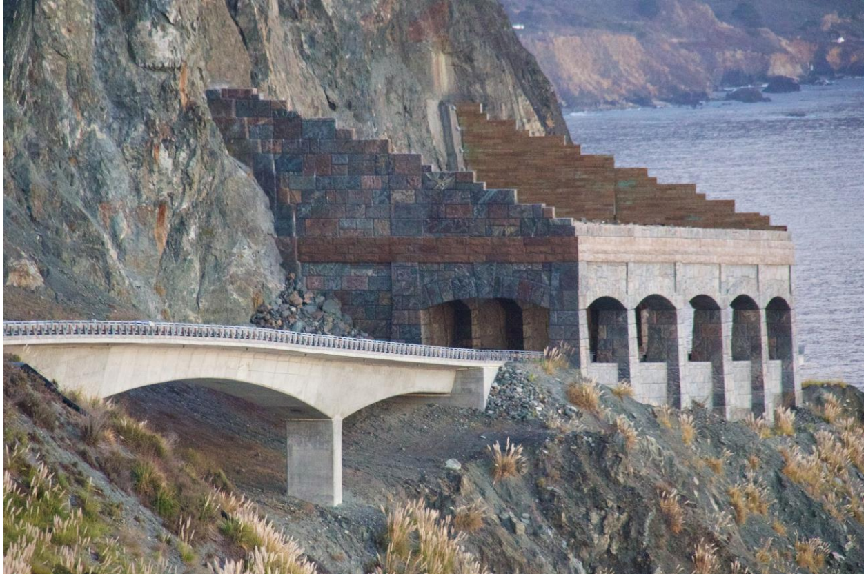
The Pitkins Curve Bridge (rocks go under) and Rain Rocks Rock Shed (rocks go over) protect Highway 1 from rock slides – at least for about 900 feet of roadway.
